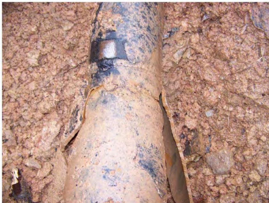
Date 1/6/09 Columbia Gas Transmission Inc. Coco Storage C field Line number X-52C-W7329 diameter 6.625 inches, .280 inch wall thickness, X-35 Description of photo – Tie in side where fracture stops at weld
