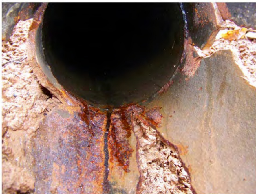
Date 1/6/09 Columbia Gas Transmission Inc. Coco Storage C field Line number X-52C-W7329 diameter 6.625 inches, .280 inch wall thickness, X-35 Description of photo – Tie in side where the fracture stops at a weld
