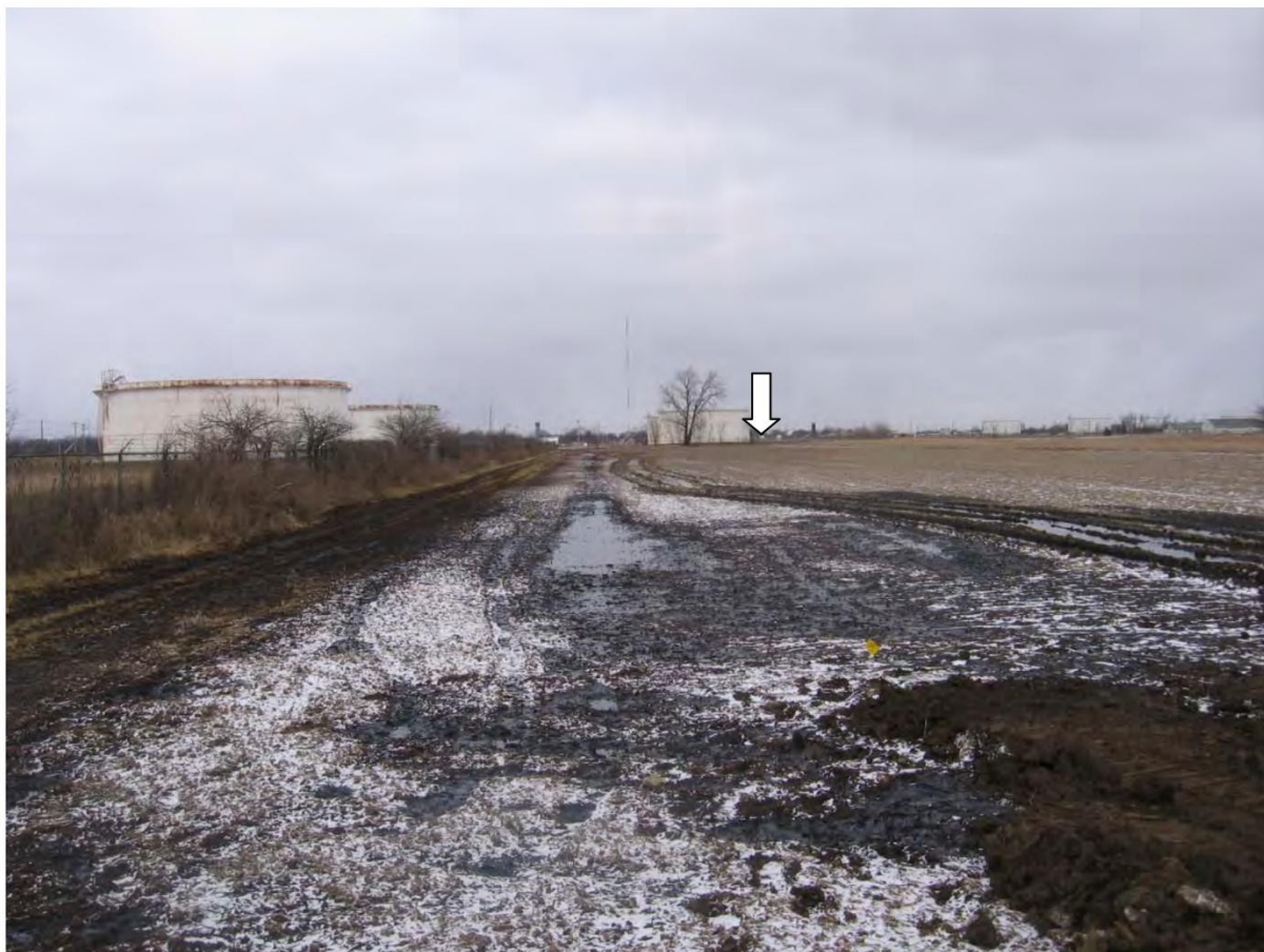
Photo 1 – View looking north from leak site. Tanks visible in the photo are no longer in service. The arrow points to Tank Farm Road.
