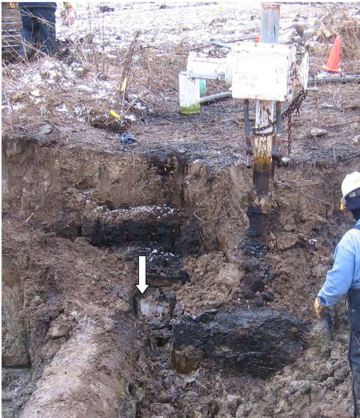
Photo 6 - The photo shows origin of the leak. The arrow points to the crack.
