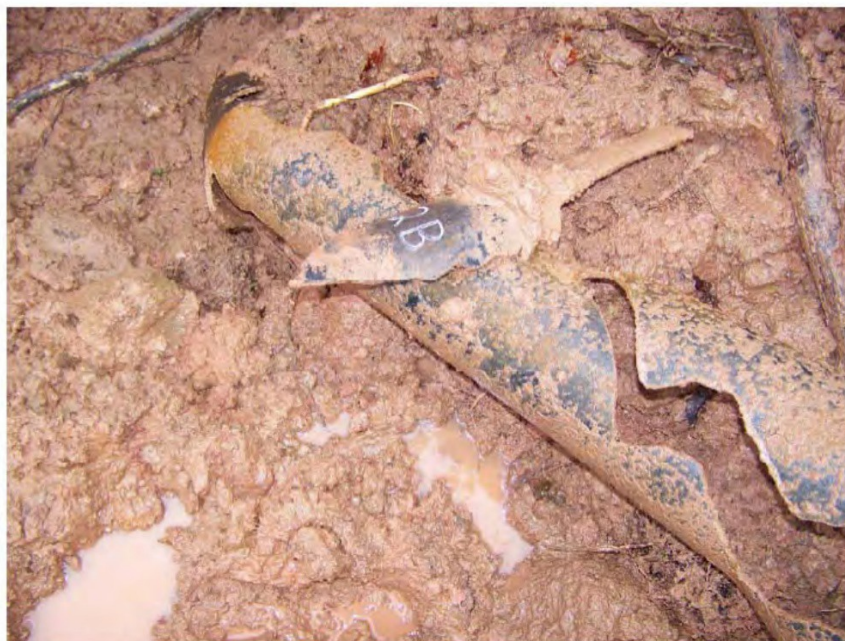
Date 1/6/09 Columbia Gas Transmission Inc. Coco Storage C field Line number X-52C-W7329 diameter 6.625 inches, .280 inch wall thickness, X-35 Description of photo – Short section of line 7329 indicating brittle fracture
