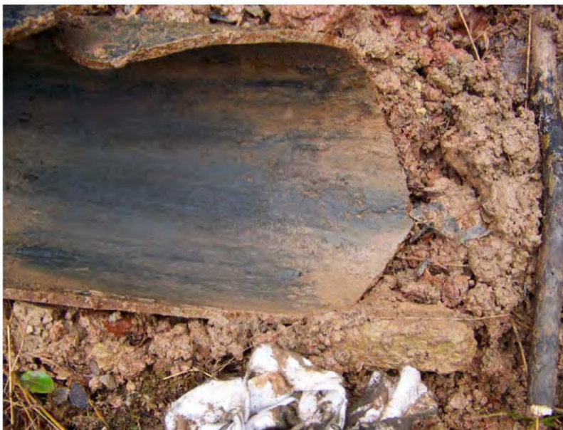
Date 1/6/09 Columbia Gas Transmission Inc. Coco Storage C field Line number X-52C-W7329 diameter 6.625 inches, .280 inch wall thickness, X-35 Description of photo – Pipeline indicates internal corrosion.
