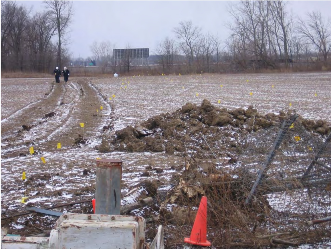
Photo 3 - The photo shows the view south of the branch connection. The tree line indicates Rocky Ford Creek. Field tile drain to the south into the Rocky Ford Creek and crude oil did reach the creek through the tile.
