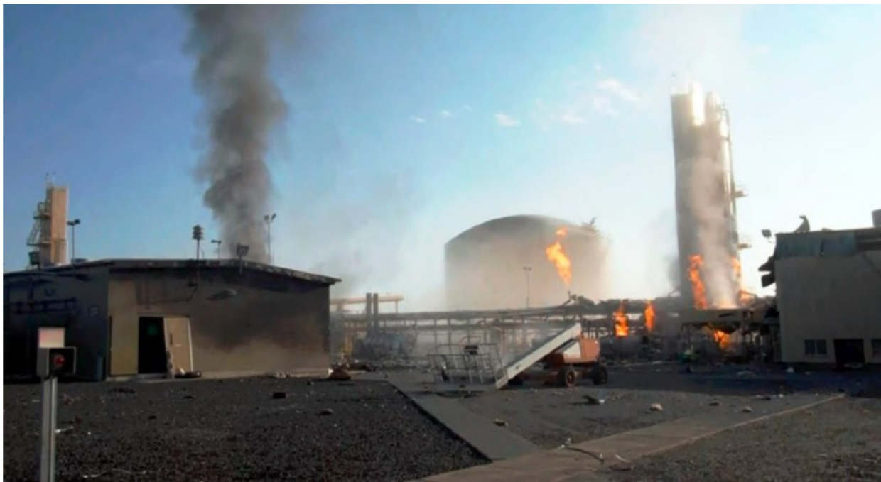
PHOTO: "A pipeline running to a Williams Companies LNG storage facility in Plymouth, Washington exploded and sent shrapnel flying that ruptured an LNG storage tank. Nearly 1,000 residents were evacuated and at least five employees at the facility were injured": http://www.sightline.org/2016/06/03/williams-companies-failed-to-protect-employees-in-plymouth-lng-explosion/
